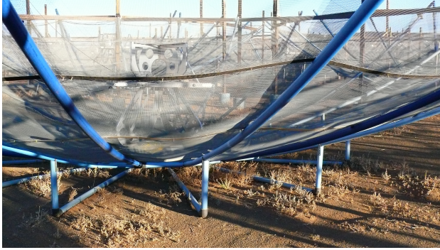
Figure 2: Mesh panels between PCV radials, if not taut, can sag and form ripples in the mesh surface.
